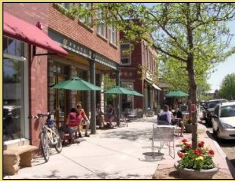
Mixed-use buildings on Belt Line Rd./Main St.
