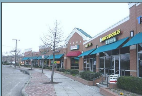
Existing multi-tenant shopping center at SE corner of Polk St. and Greenville Ave.
