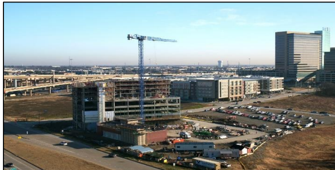
Construction underway on the Drury Inn &amp; Suites Hotel
