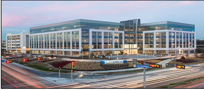
Completed Transwestern five-story building
