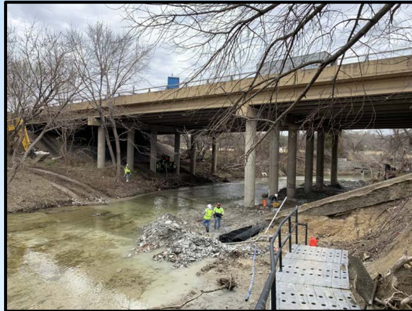
Jupiter Road Bridge Slope Stabilization
