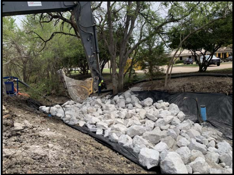
Nantucket Branch Channel Improvements
