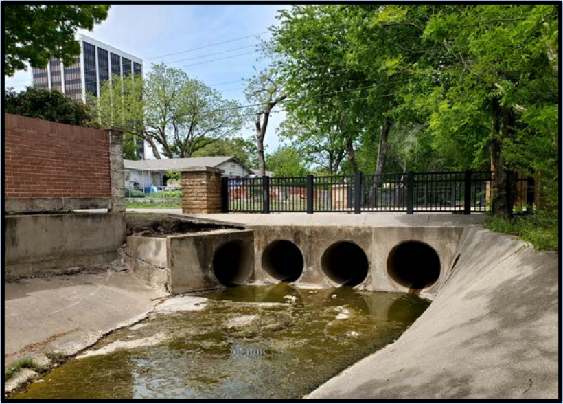
Hunt Branch at Cherrywood Drive Culvert
