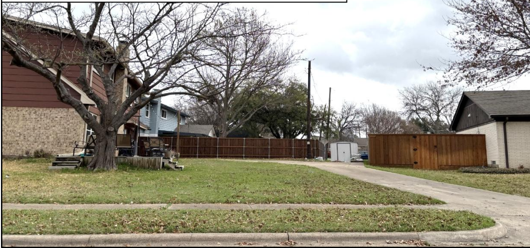
West Elevation – View from Sandalwood Avenue
